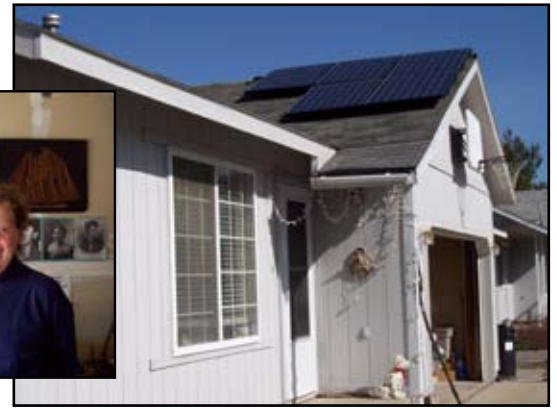
Above: Warner's home with the panels installed. Left: Warner stands next to the controls in her garage.
