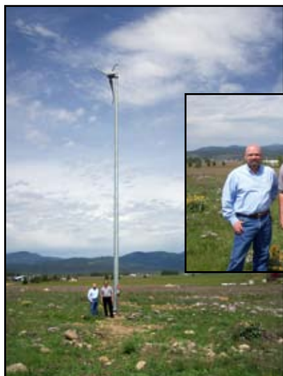
Above: Mark Gibson, Project Manager for Wind2Energy.Net, left, and Steinbach, right, stand next to the wind generator and switch.
